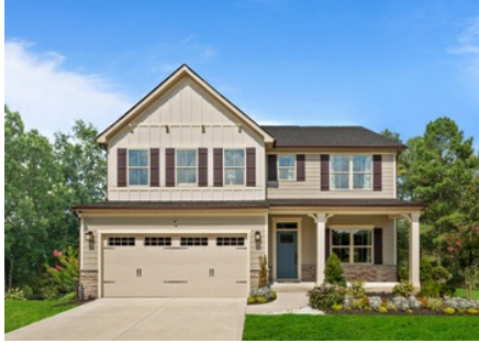
Creekside Crossing By Ryan Homes
